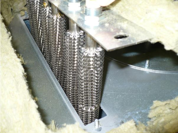
9. Replace Heater- If bad – check heater for continuity with wires removed
