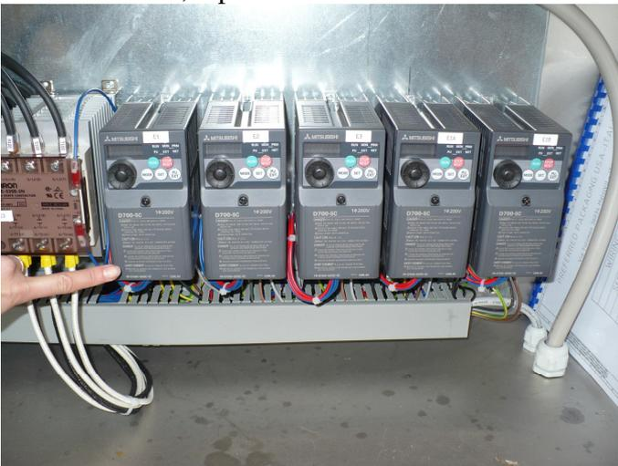
3. Check solid state relays KS1 and KS2, check if voltage is present at -4 and 3+ (10 volt DC need to be present)
